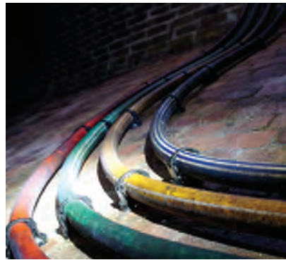
Geo extended its fibre network by three kilometres through London's sewers to reach DataRoom's data centre at Woolwich Arsenal.
