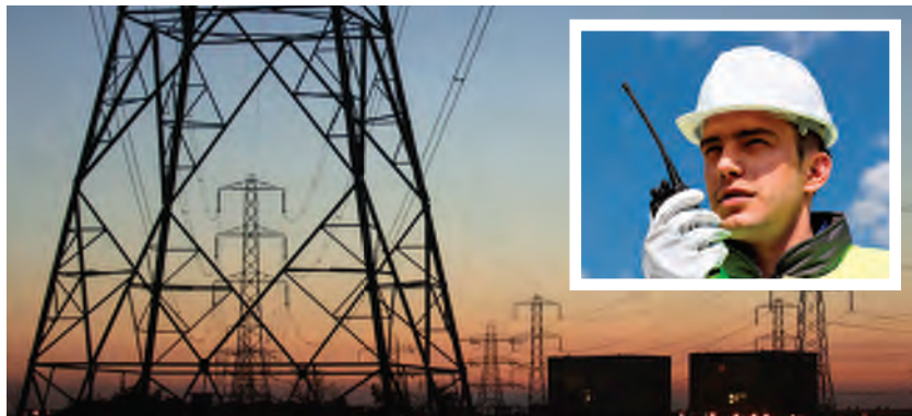
Simoco PMR proved more reliable – and therefore safer for staff – than cellular in severe weather.
