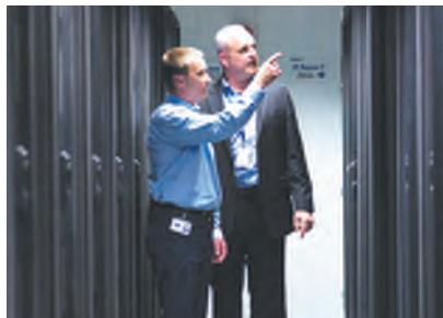
Engineers inspect TalkTalk Business' racks at Ark Continuity's new Corsham data centre.
