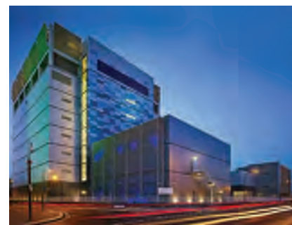
Based in London's East India Dock, Telehouse West offers 5,000m 2 of colocation space and power capacity between 2 to 10kW per rack.
