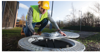
Vodafone UK's senior networks manager Mohamed Elhabiby installing a 4G-enabled manhole and cover in Newbury, Berkshire. By connecting manhole covers to its all-fibre fully converged network, Vodafone says it can provide improved 4G coverage today as well as future 5G.
