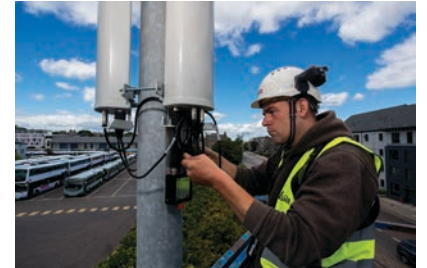
An engineer installs a small cell radio for O2 on a lamppost in Aberdeen.
