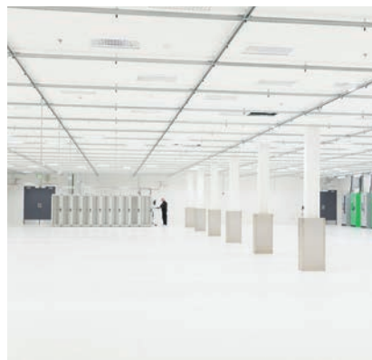
VIRTUS operates two Tier 3 data centres – LONDON 1 in Enfield and LONDON 2 (pictured), its new, 65,000ft² flagship facility in Hayes.
